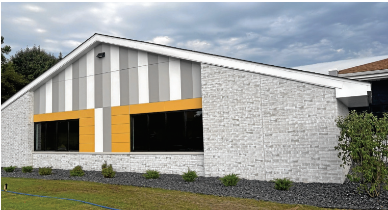
Shoreland Lutheran High School recently completed its $7.3 million expansion project with a new atrium, new classrooms and more. The school hosted a community ceremony on Sept. 3 to celebrate the milestone.
